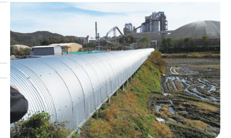
Limestone belt conveyor
