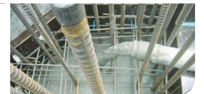
Photo of ultra high-strength Cement/concrete placement
