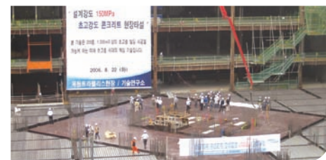
150MPa ultra high-strength application to site
