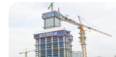
Photo of ultra high-strength Cement/concrete applied
